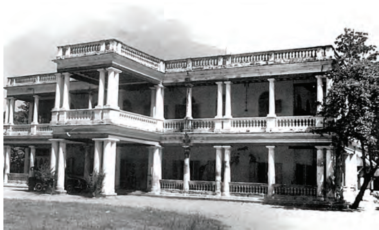
Fig. 12.18 A garden house on Poonamallee Road
